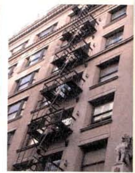
6 a fire escape
